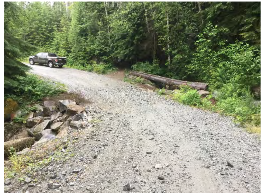
Approach from Left Bank when facing downstream
